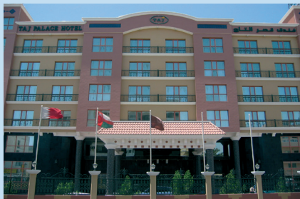
TAJ PALACE HOTEL ISSA TOWN 2 units of 1500L calorifiers
