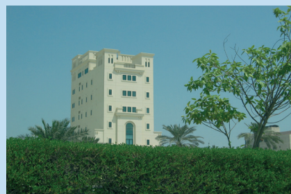
TARIQ HOSPITAL 39 units of 1500L calorifiers
