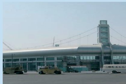
AL SAAD SPORTS CLUB DEVELOPMENT 10 units from 1000L to 3000L calorifiers
